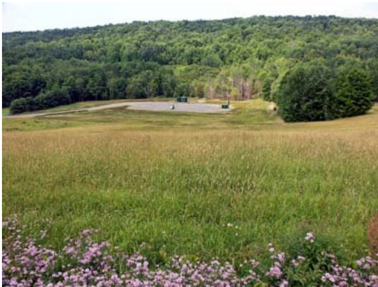
An active natural gas well in Chemung County after the drilling and completion work is done and the site has been reclaimed. Courtesy of NYSDEC.
