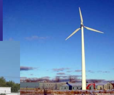
Harbec Plastics Ontario NY 250 kW Fuhrlander FL250, 213 feet total height
