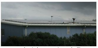
The intent of the project was to zero out electrical consumption at the Town garage by installing 144 solar panels and a 3-phase utility interactive inverter. Since the system became operational in early May 2011, there has been a decline in power bills during the months of May, June and July. It will take approximately a year for the Town and National Grid to review the Town's electric usage post construction.
