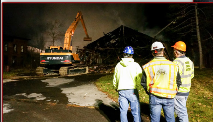
Vanduzee Street Warehouse Fire /Asbestos Site Cleanup City of Watertown
