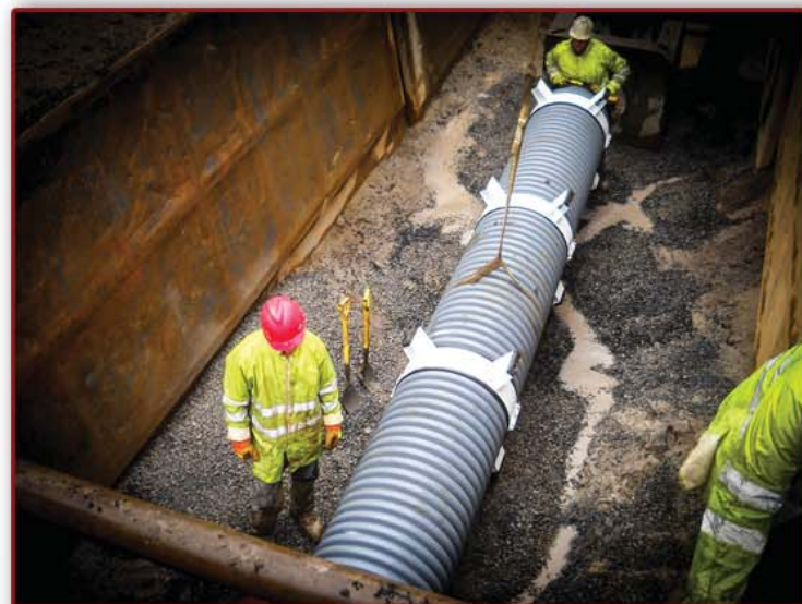
Installation of a 24" sanitary line in a 48" casing being part of the Sanitary Sewer Conveyance Project in the Village of Lowville for the Kraft Plant.
