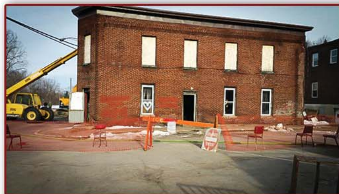
North Mechanic Street Demolition Project Village of Carthage
