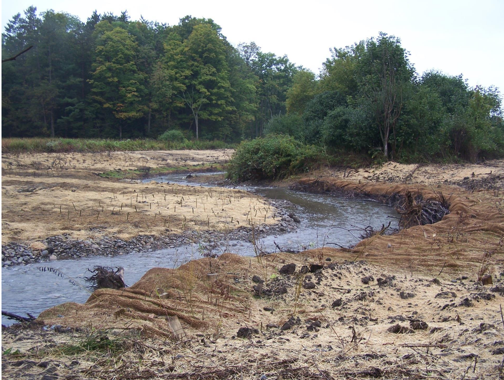
Facing downstream from the meander toe wood in September of 2016 approximately 1 week post construction.
