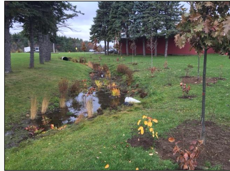
County highway facility bioswale
