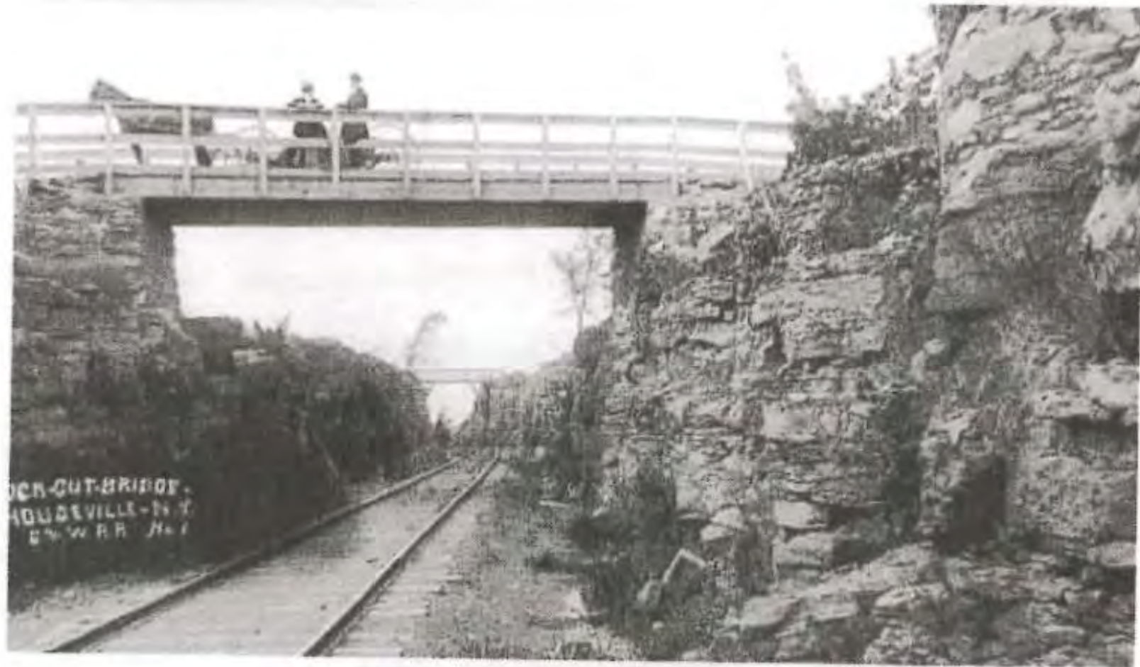
Rock Cut & Bridges Near Houseville
