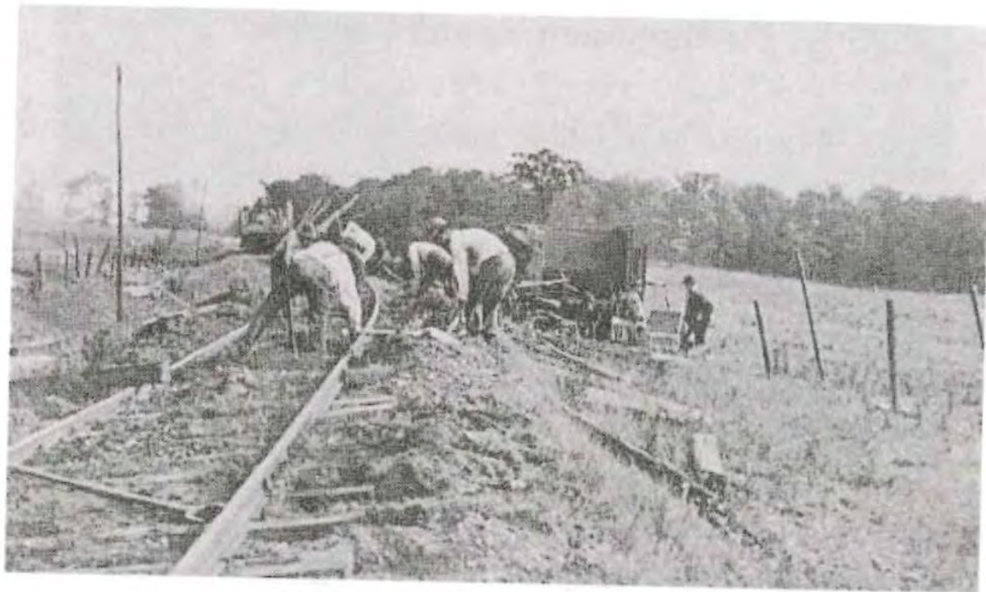
Repairing Tracks at Bardo's Crossing
