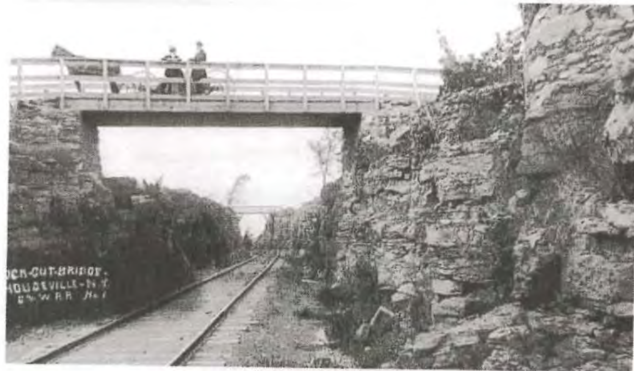
Rock Cut & Bridges Near Houseville
