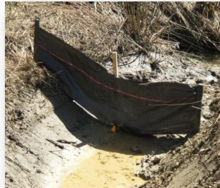
An example of ineffective erosion control practice – silt fencing should be buried to a depth of about 8 inches. Also, silt fencing is not intended for use in drainage ways.
