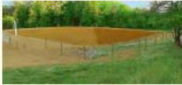
Construction of an agricultural waste system.
